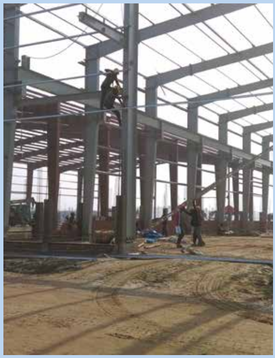
Ware House Construction
